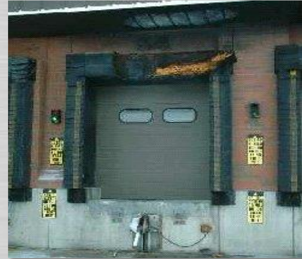
"It took three fire extinguishers to put it out! We're lucky the whole building didn't catch fire." - Shipping Manager, CWC Textron
