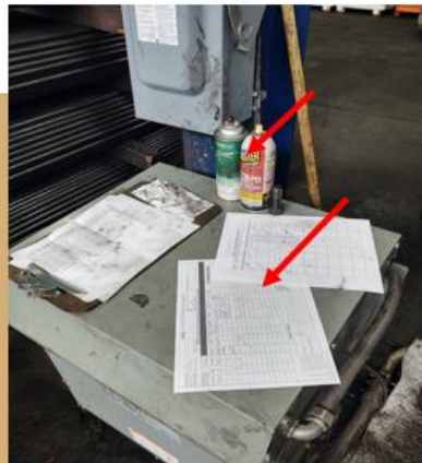
Using a transformer as a paper shop desk. Also unsafe storage of spray cans
