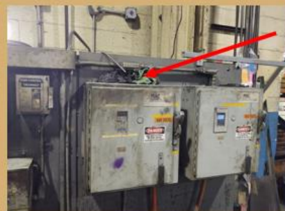
Unsafe storage: Rags on top of electrical box
