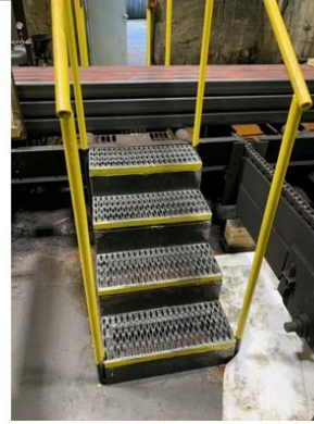
Handrail added and diamond plate stairs replaced with treaded stairs
